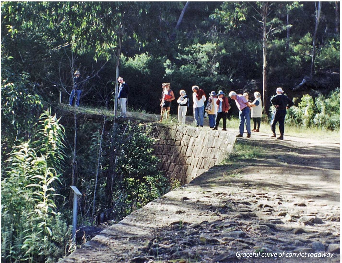
Devine's Hill roadway
